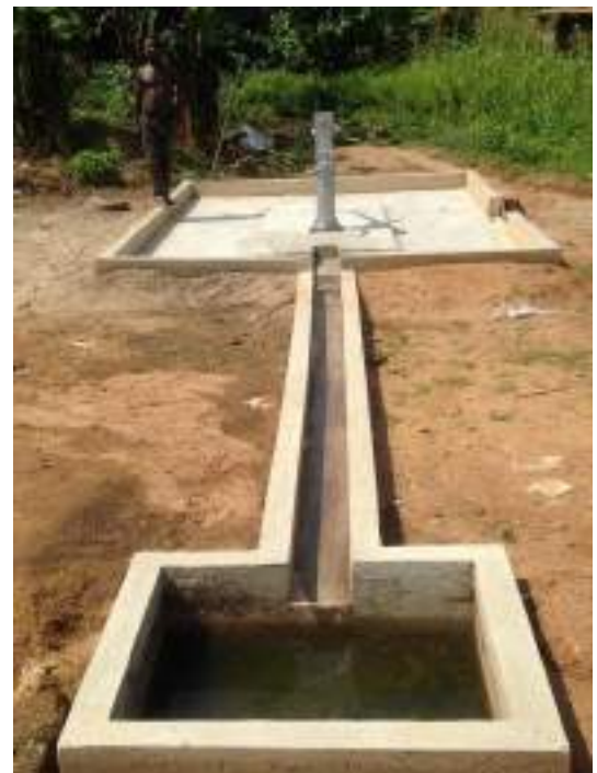
Photo Above: Repaired pump with a new concrete pad in Sunyani West District.
