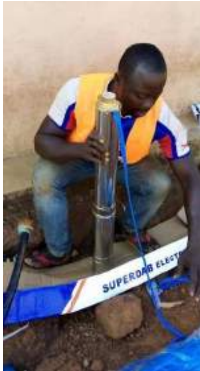
Left & Center: Replacing electric pump for mechanized pump at Mpuasu and water flowing from fetch point under water polytank. Right: Water flowing again at Anunguano 1.
