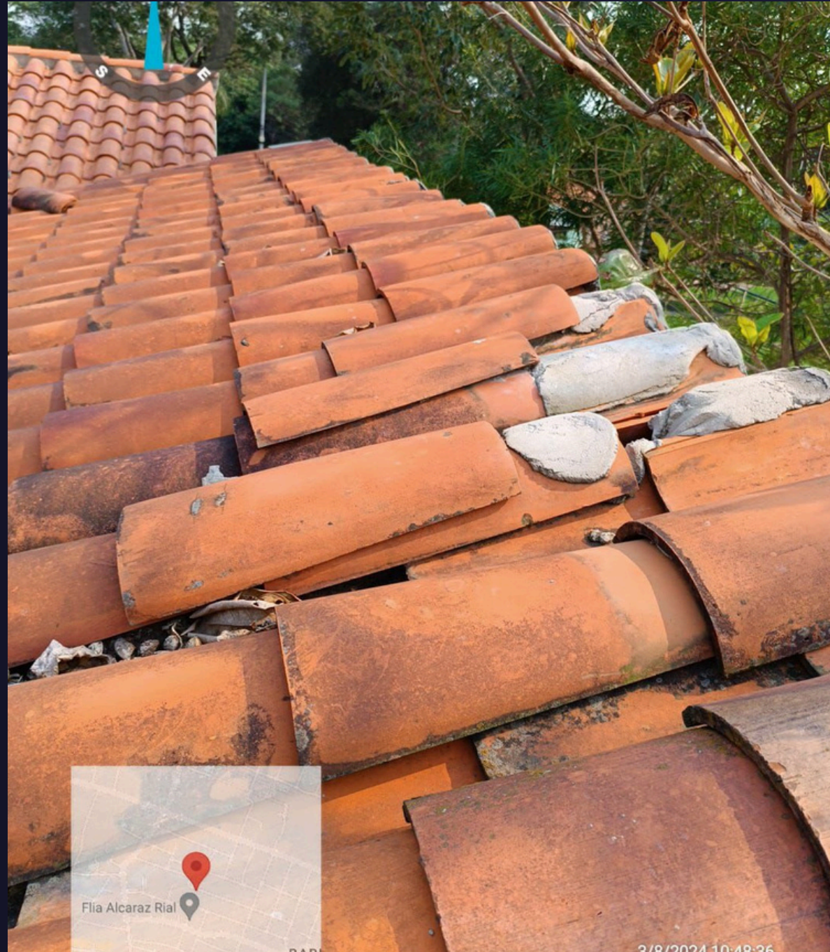
Ceiling showing signs of damage
